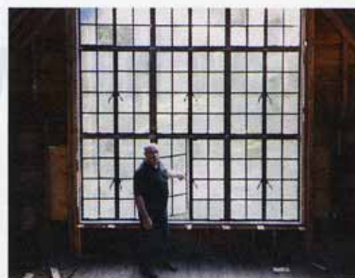
Seekircher restores steel windows in residential and commercial buildings.
