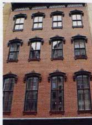
The double-hung windows of this building were custom designed by Parrett Windows and installed with weight-and-pulley sash and balance systems.
