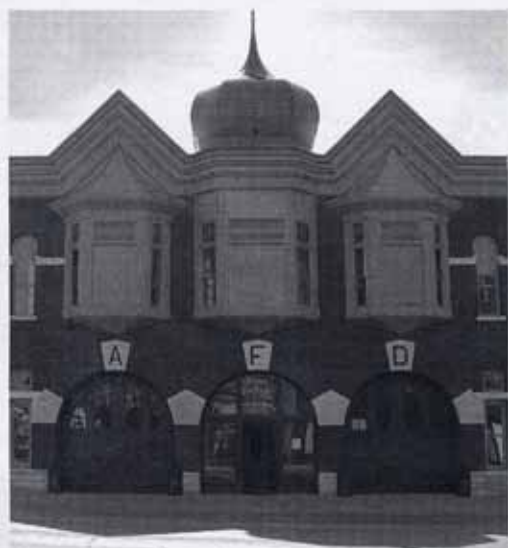
Richards-Wilcox replicated the traditional hardware for the restoration of the Aurora Fire Museum in Aurora, IL.
